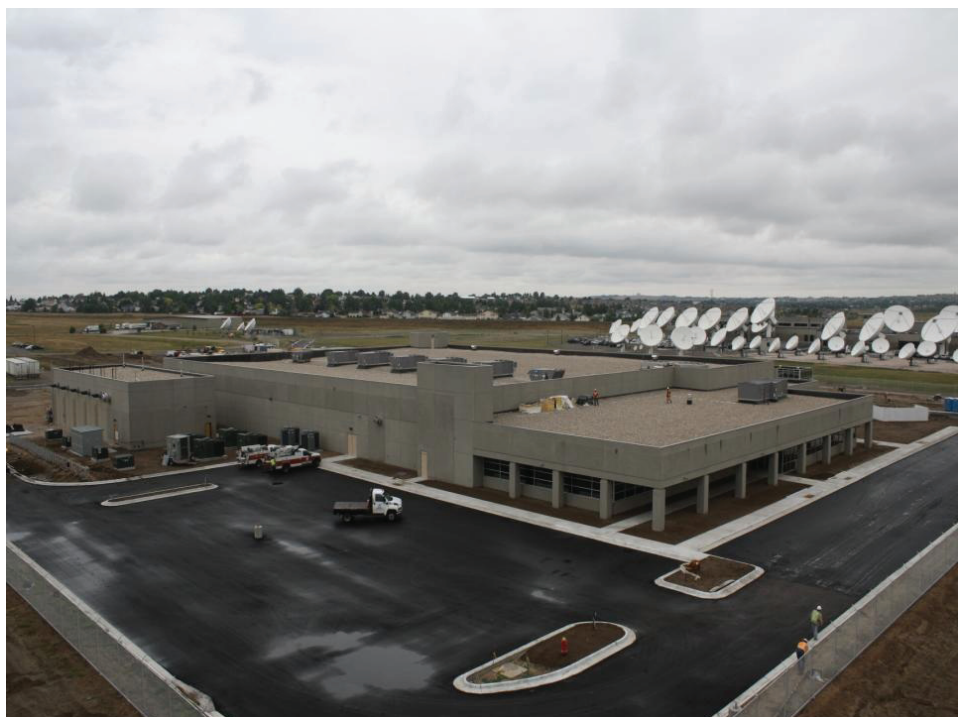
This recent photo shows the Cheyenne Datacenter for EchoStar Broadcasting Corporation adjacent to their existing facility in LEADS Cheyenne Business Parkway. (Photo courtesy of EchoStar Broadcasting Corporation)
